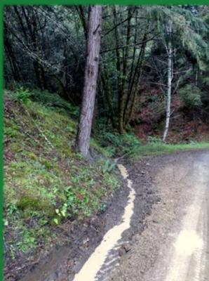
Conduct all road recontouring and grading during the dry season, if possible. Excavation in the winter promotes surface erosion that can be washed into nearby streams.
