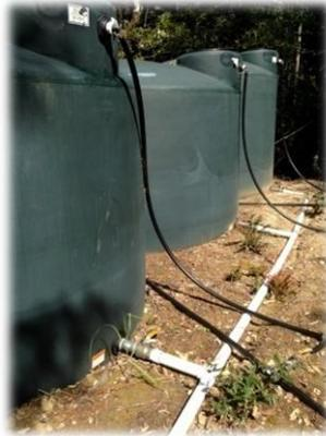
Whenever multiple tanks are installed for water storage, each tank should be equipped with its own shut off valve. This prevents catastrophic loss of water, if one valve in the system is left open.
