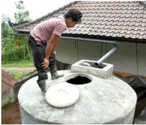
Rain water from your roof can supply a significant amount of the water you use. If your roof is plumbed into a storage tank, you can get 600 gallons of water from every inch of rain per 1000 square feet of roof. Water use and storage in this way does not require a permit from any agency.
