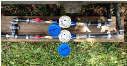
You need a water meter that measures domestic and garden use separately to understand your water needs and to do a water budget. Make sure that you purchase a system with a leak indicator to prevent unneeded loss and water waste.
