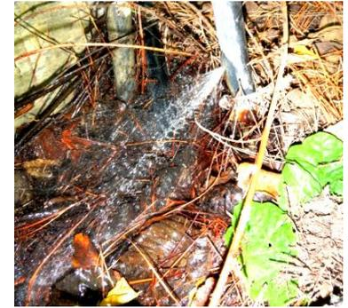
To check for leaks, turn off the supply to your home and garden. If your meter is still running, find and stop your leak immediately. Install a float valve in your tank to prevent over-flow. Leave as much water as possible at the source.
