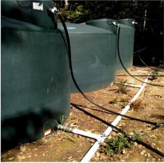
Water storage can increase water security and decrease the need to draw from streams when fish need it, but you need to do a water budget to know how much storage you need. Collecting roof runoff does not require a permit. You can catch 600 gallons per 1000 sq feet of roof from only 1 inch of rain! Even if you have an ample water supply, roof catchment is a good thing to add.
